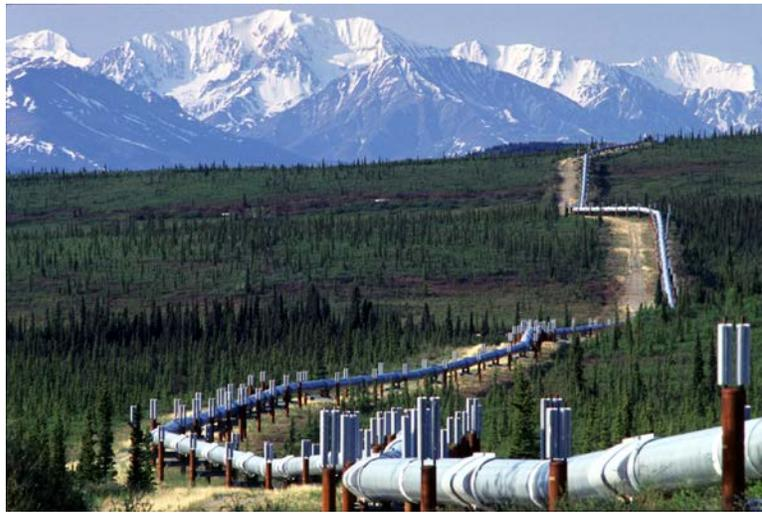
To help move the oil along the pipeline, 12 pump stations were installed. Pigs, or mechanical devices push through the pipeline. They improve the flow characteristics (scraper), inspect for dents and wrinkles, inspect for pipeline corrosion, and measure pipeline curvatures.
